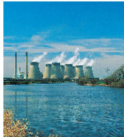
Figure 10 This power plant uses cooling towers to cool the warm water produced by the power plant.
