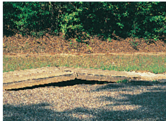
Figure 2 Most objects expand as their temperatures increase. Pieces of this concrete sidewalk forced each other upward when the concrete expanded on a hot day.
